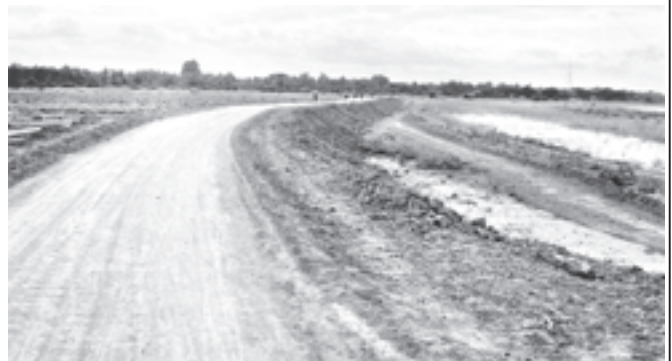
Progress in ground work of Yesagyo-Tamadan embankment.
