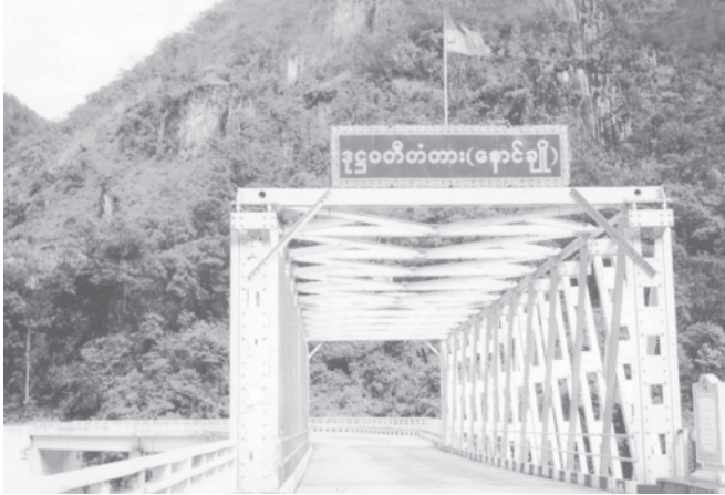
Dokhtawady Bridge (Nawnghkio in Shan State (North)).
