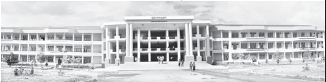
Three-storey main building of Loikaw University.
