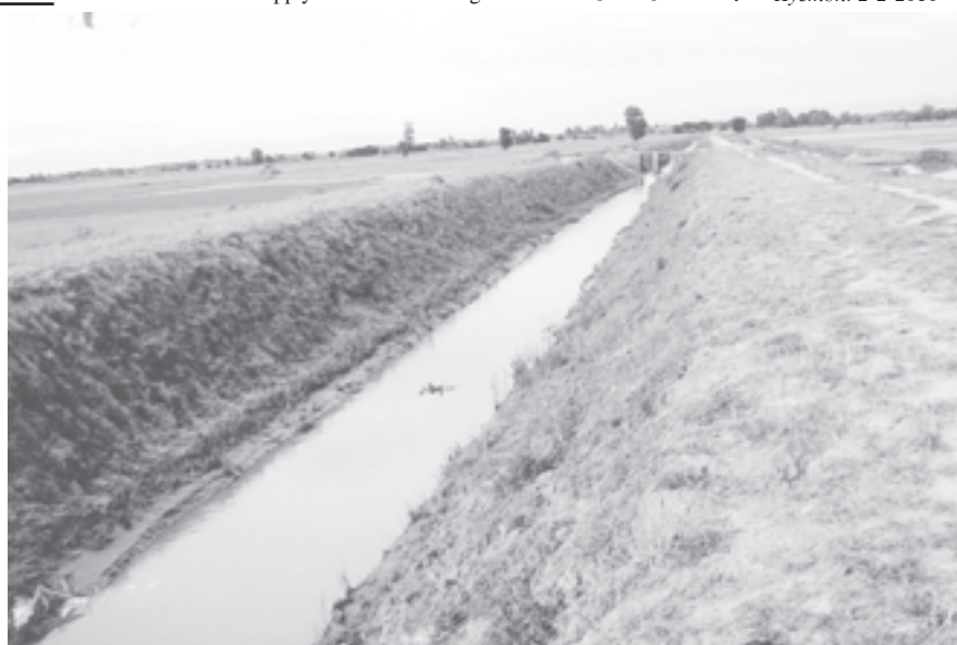
A canal of Chaungmange Dam.
