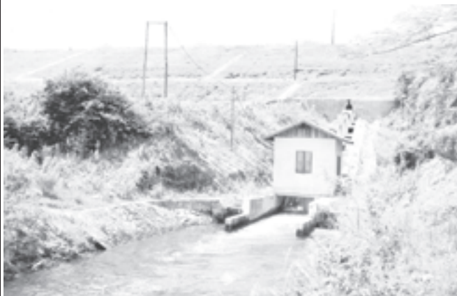
A small-scale hydropower plant at embankment of Chaungmange Dam to supply power to nearby villages.
