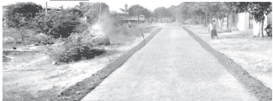
Industrial Zone (1) Road is in the process of being upgraded.
