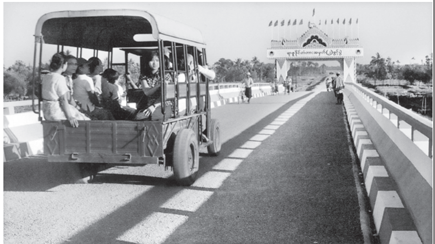
A group of people in a car passing through the newly-opened Yazudaing Bridge No. 2.
