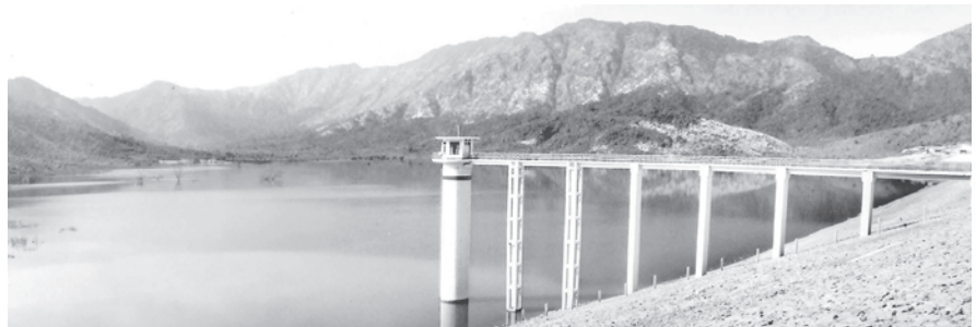
Kadaik Dam contributing to regional development.
