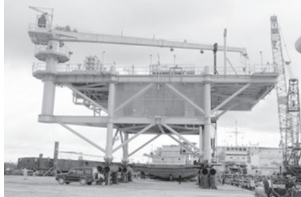
An oil platform on the outskirts of Port Harcourt. The Nigerian government is in talks with the United States oil firm Chevron and Anglo-Dutch oil giant Shell over the renewal of their shallow water oil licences, an official statement said on Tuesday.—INTERNET
