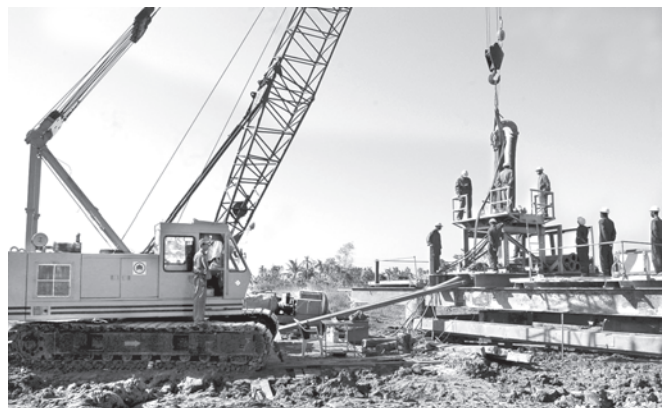
A heavy machinery unit driving a bored pile for Yazudaing Bridge No. 1 in Mawlamyinegyun Township.
