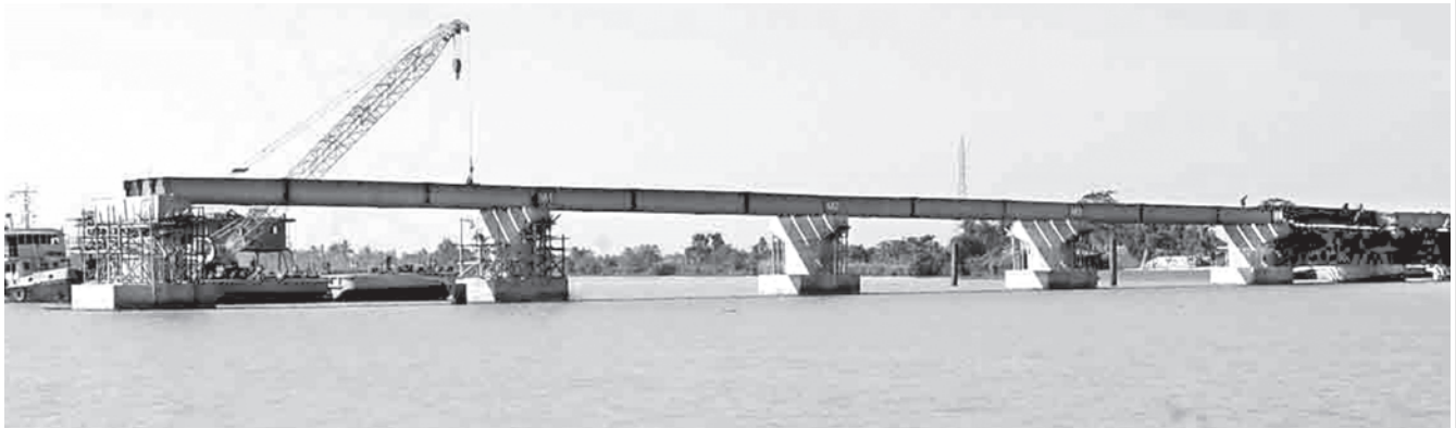
Ongoing construction of Yazudaing Bridge No. 1.
