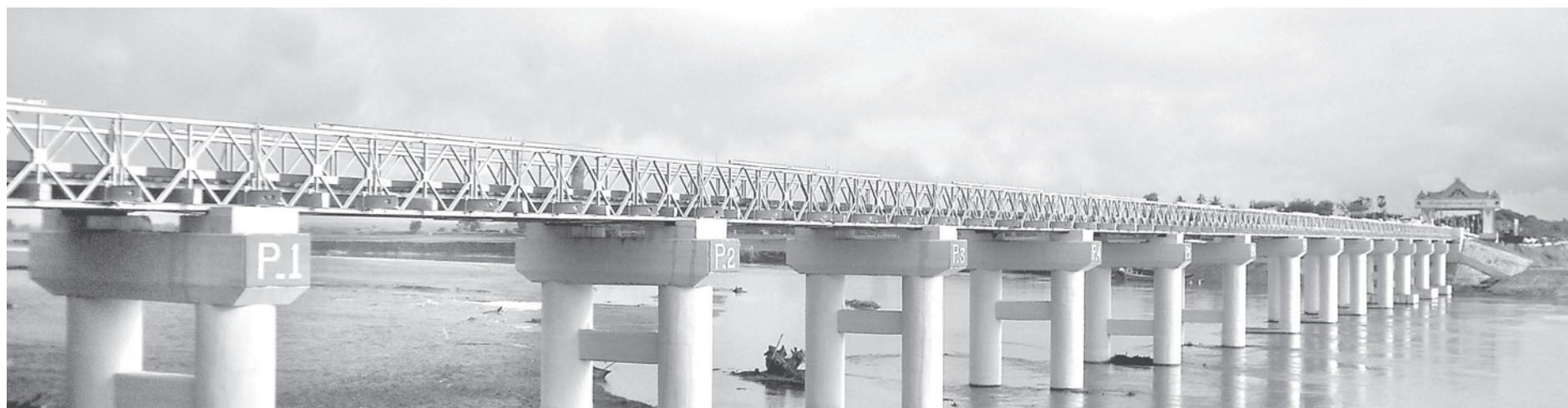
Mindon Bridge (Yenatha) in Kanma Township of Magway Division.
