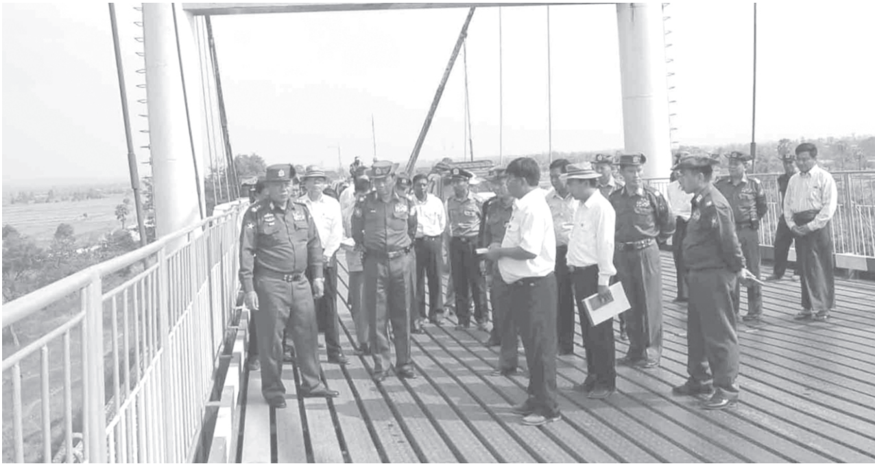
Lt-Gen Khin Zaw inspects maintenance of Gyaing (Kawkareik) Bridge. (News on page 16)—MNA
