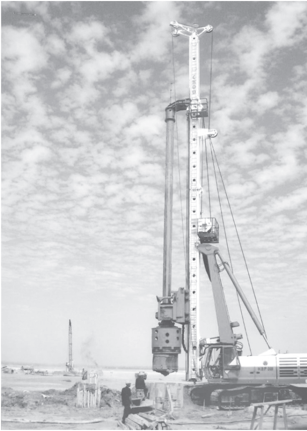
A heavy machinery unit driving a bored pile on Letpanchepaw side in Ayeyawady Bridge (Pakokku) Project.
