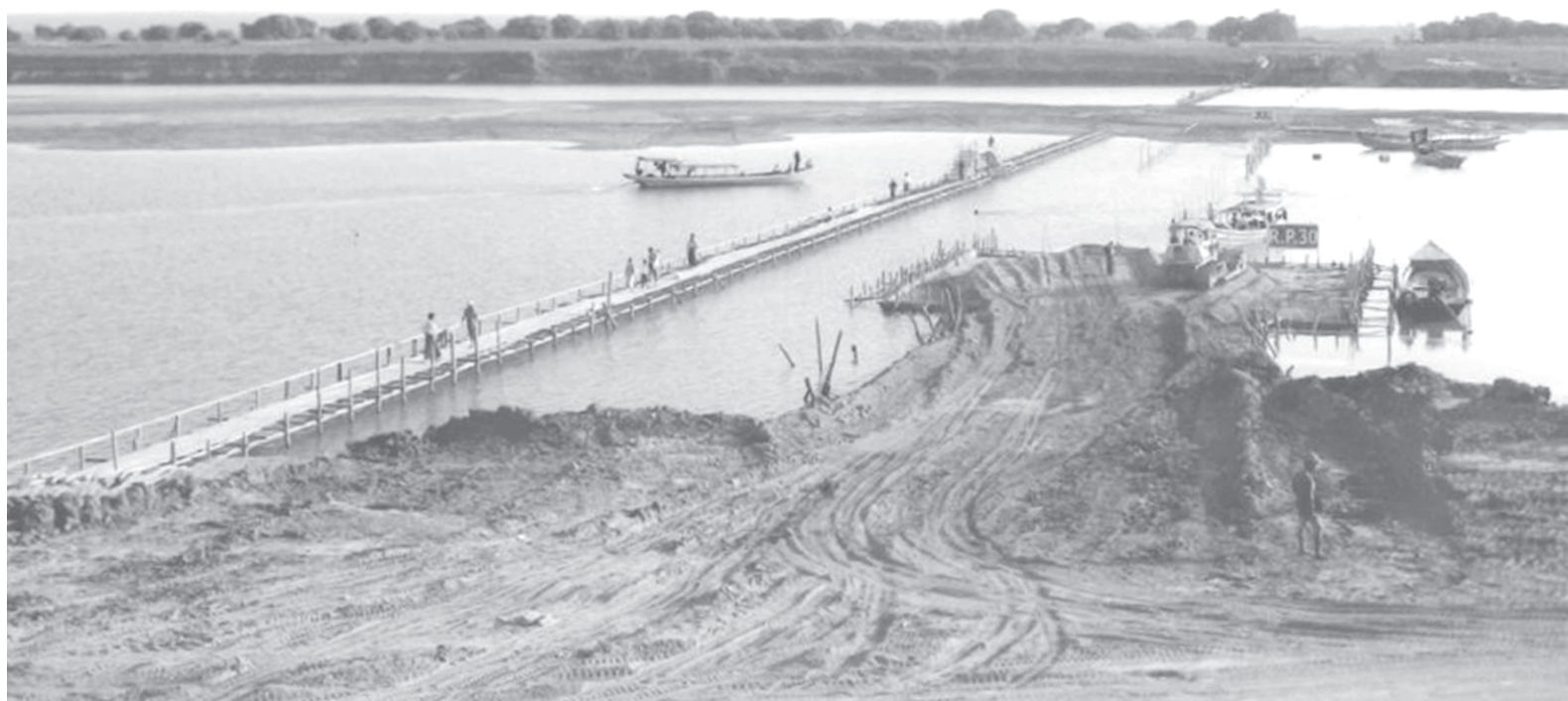
Groundwork in progress to drive RP 30 and RP 29 bored piles.
