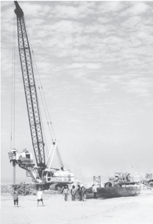
The construction site on Letpanchepaw side in Ayeyawady Bridge (Pakokku) Project.
