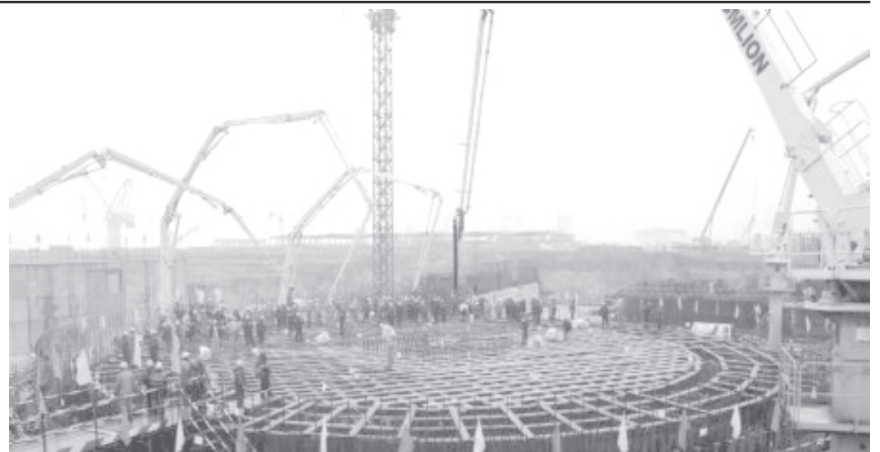
Photo taken on 8 Jan, 2010 shows the construction site of the third generator of the Ningde nuclear power plant in Ningde, southeast China's Fujian Province. Ningde nuclear power plant, the first in Fujian, started building its third generator Friday. With an investment of 50 billion yuan (6.8 billion US dollars), the Ningde plant would be equipped with four 1-million-kilowatt generators in the first-phase construction. Its first generator would be installed in 2012. —XINHUA
