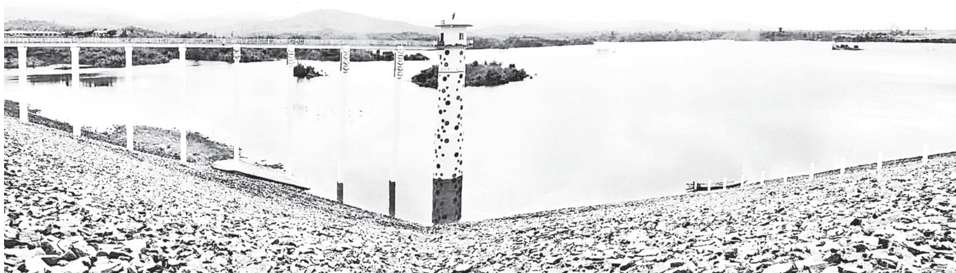
Photo shows Ma Mya Dam and its control tower.
