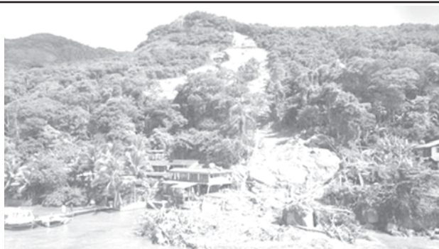
An aerial view of Pousada Sankay hotel buried by a mudslide in Angra dos Reis, Rio de Janeiro state on 1 Jan, 2010. —XINHUA
