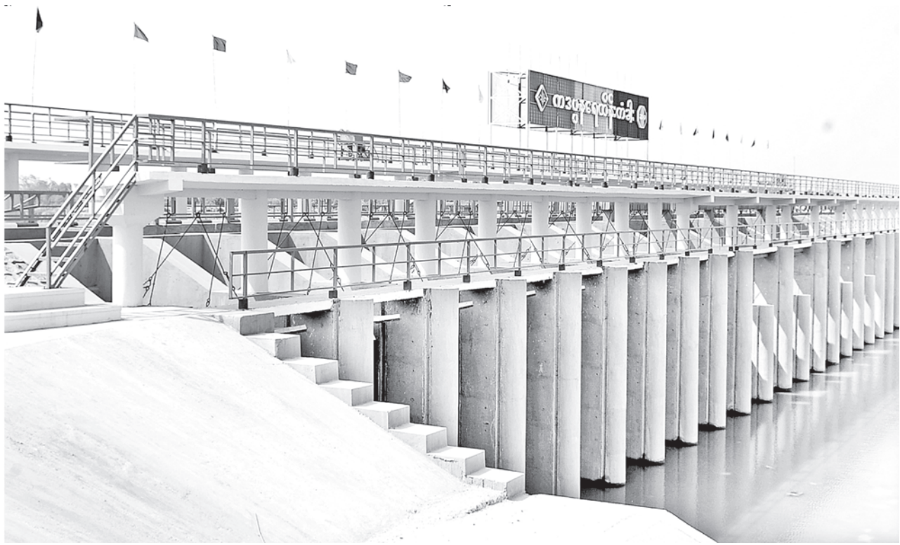
Kadatpana sluice gate near Katatpana village in Kyauktan Township, Yangon Division.
