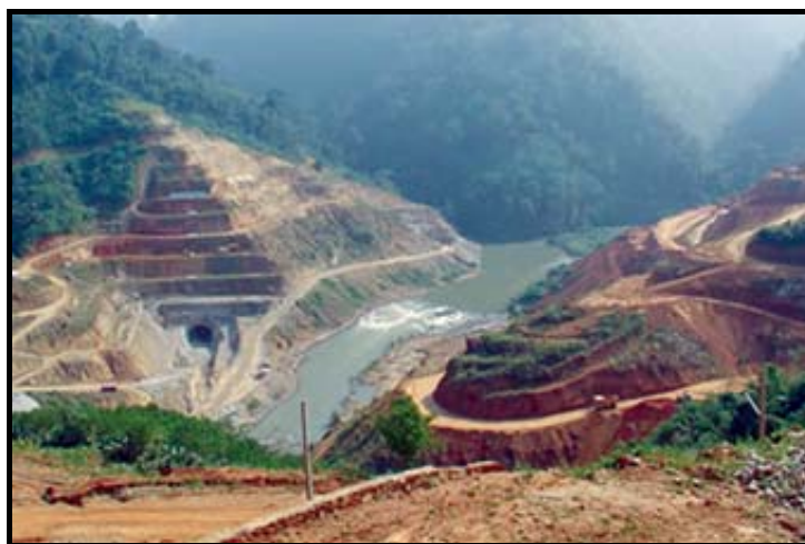
The site of the Upper Paunglaung Dam in Karenni State. Rights groups have estimated that the construction of the dam will inundate at least 12 civilian villages and displace an estimated 3,500 people. [Photo: © YMEC]
