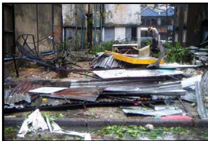
Debris littered the street of Rangoon in the wake of the cyclone. Roofs were ripped from houses, while trees were torn from the ground. Anything less structurally sound was simply destroyed. [Photo: © Mizzima News]
