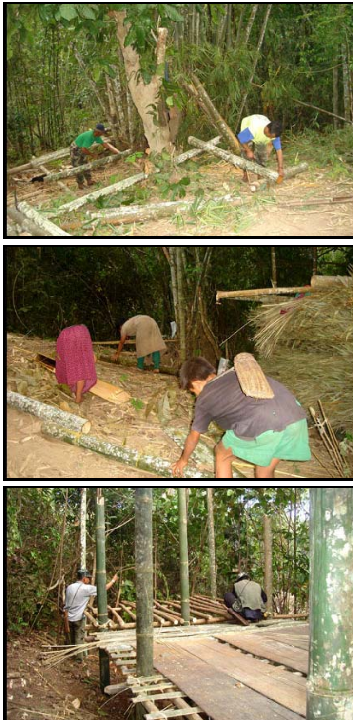
Civilian villagers from Bpo Gkweh village in Karen State rebuilding their homes in the forest after SPDC army soldiers had attacked them and driven them from their homes at the end of 2007. Villagers in northern Karen state are often displaced as a result of military activity and have become quite skilled in quickly establishing new hiding sites and constructing new shelters out of locally available materials such as bamboo and palm thatch as can be seen in these photographs. Despite their circumstances, these villagers are able to maintain a semblance of ordinary village life and live with dignity. [Photos: © KHRG]
