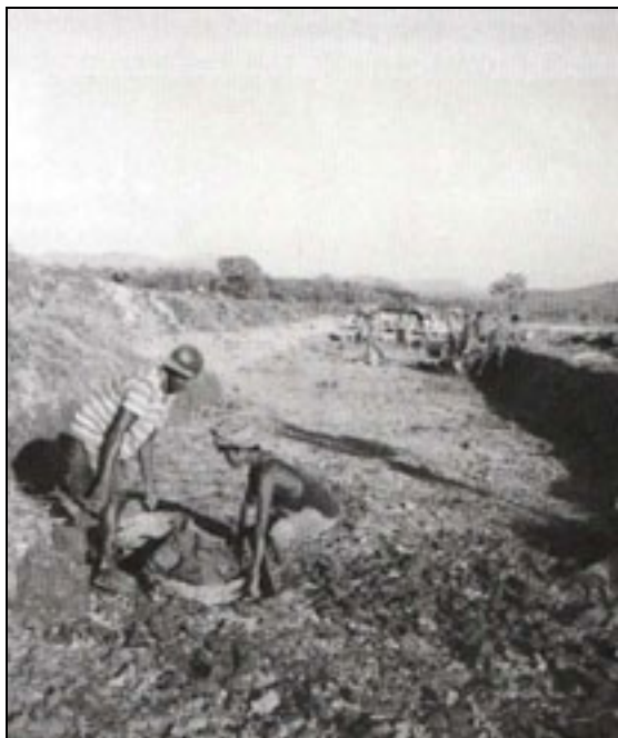
(12) Forced labour in water canal construction in Mudon township, Mon State (Photo: HURFOM) (Left)
