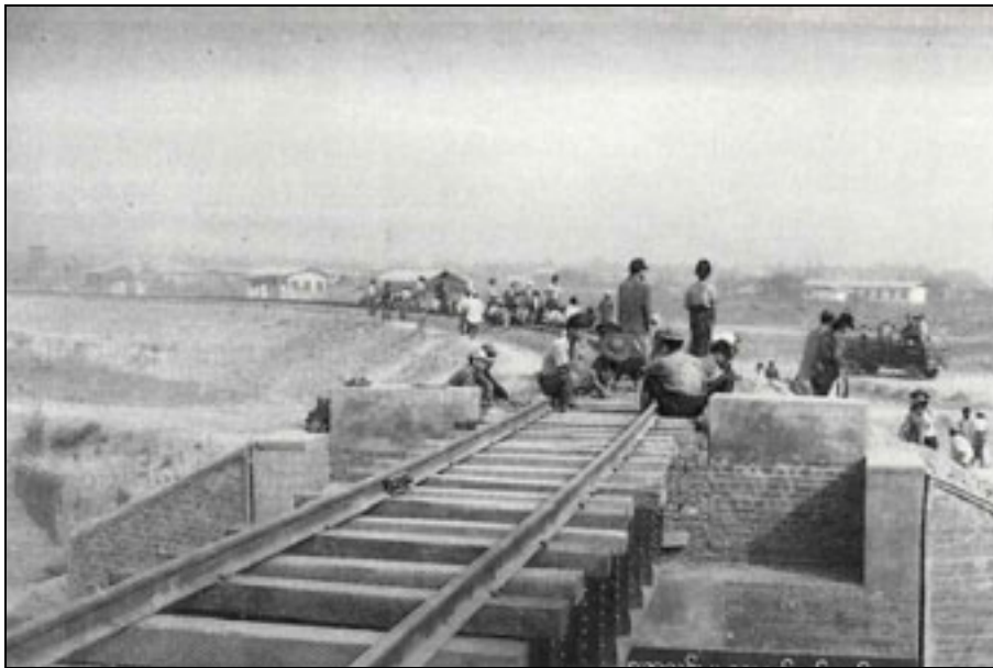
Civilians are working on the Kalay-Gangaw railway construction project in Sagaing Division. (Photo by Tarzan Htun)
