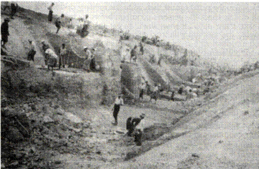
Corvee labourers from different villages in Kalay Township contributing labour for the construction of Kalay-Gangaw Railway. (photo: ABSDF)
