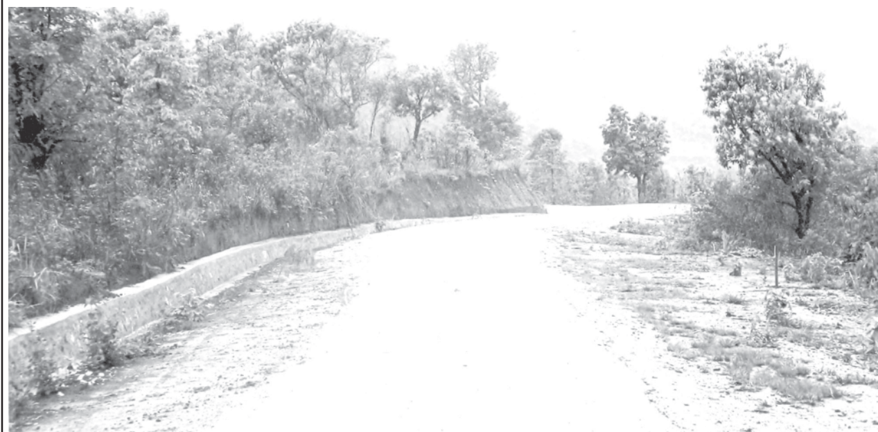
Takaw-Maipyin-Kengtung road in Shan State (East).
