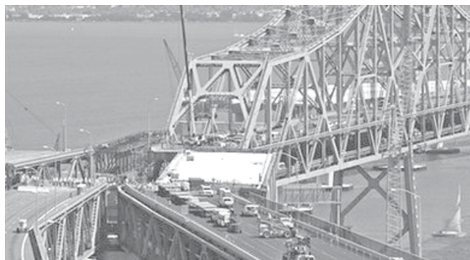
A replacement section slides into place connecting the new detour route during the San Francisco-Oakland Bay Bridge seismic retrofit in San Francisco, on 5 Sept, 2009.—INTERNET
