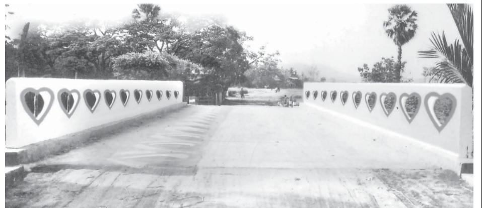
A concrete bridge on district-to-district road No.2 in The-ein village of Paung Township.
