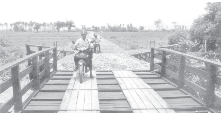
Thayetthopin-Kungyangon motor road in use.
