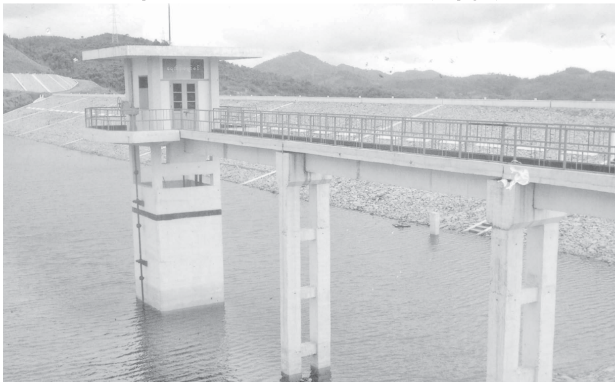
Control Tower of Sitha Dam.
