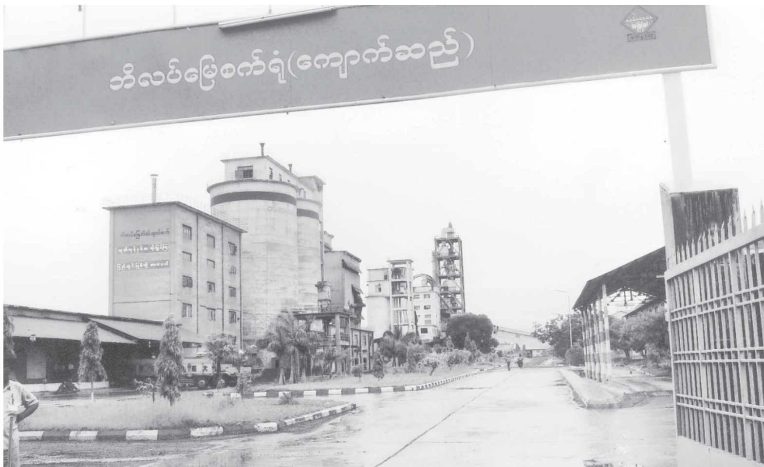
Cement Plant (Kyaukse).
