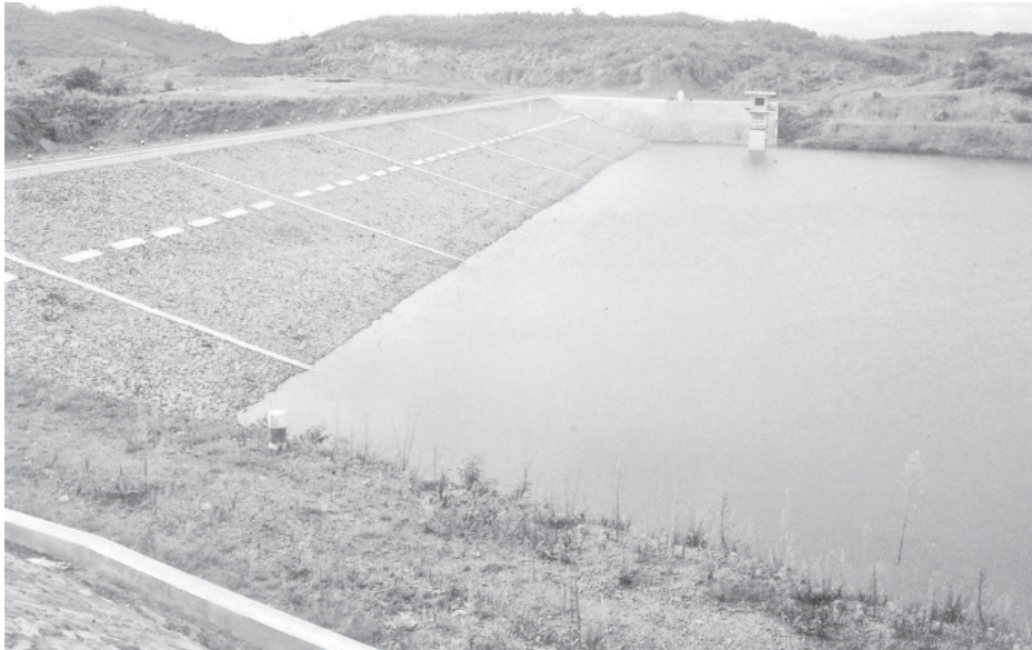
Water flowing into Sitha Supporting Dam.
