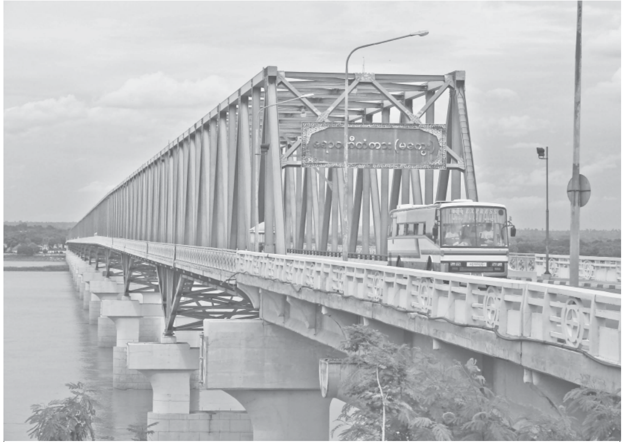
Ayeyawady Bridge (Magway) is seen from Minbu side.
