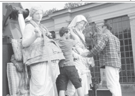
Workers at the Sanssouci Palace in Potsdam near Berlin prepare two statues that are to return to their original place on the façade of the orangery. After years of restoration, the two sculptures along with 10 others have now been put back within the magnificent palace garden. The statues depict scenes ranging from the four seasons to the sciences and were made in the 19th century.
