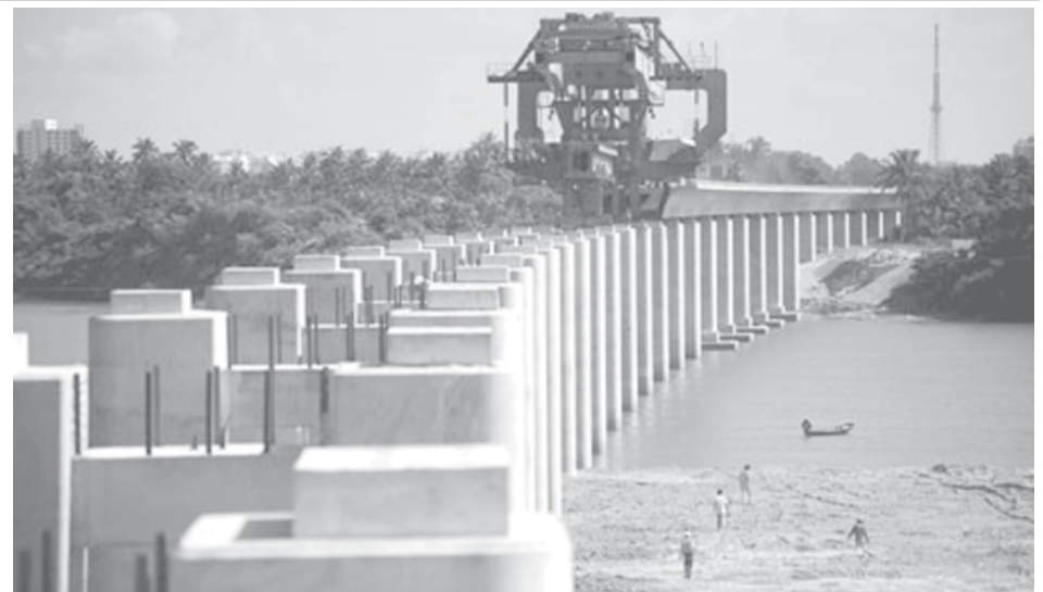
Box girders of the East Loop Railway are being installed at the work site of Wanquanhe Bridge in Qionghai City of south China's Hainan Province, on 22 Aug, 2009. A total of 122 box girders needed to be installed on the 3974-meter-long Wanquanhe Bridge, a section of the East Loop Railway of Hainan Province, which was started in Sept. of 2007 and planned to be completed in late 2010.—XINHUA
