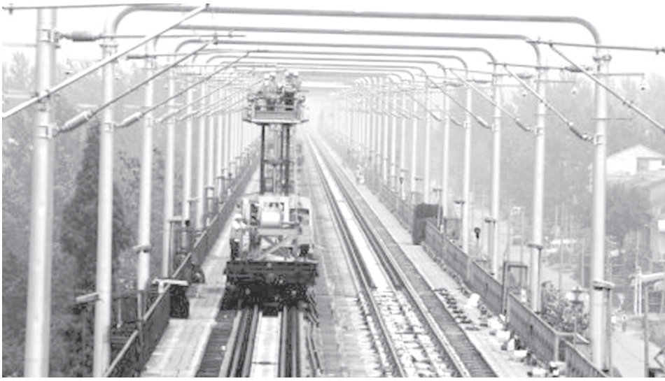
Chinese railway workers install power-transmission cables on supporting poles at the Yangtze River Bridge section of the Beijing-Kowloon Railway near Jiujiang city in east China's Jiangxi Province, on 21 Aug, 2009. The speed of the Beijing-Kowloon Railway will increase to 200km from the present 160km per hour after it is electrized.—XINHUA
