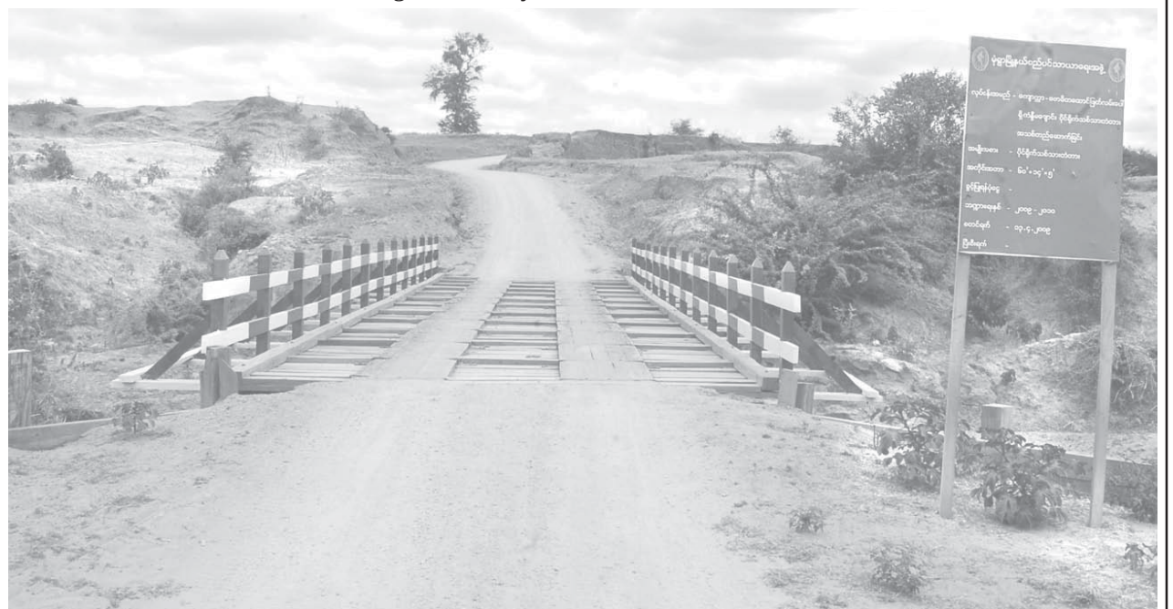
Kandima Creek bridge on Kyaukka-Bodhi Tahtaung shortcut.
