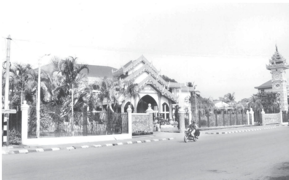
Newly-built Town Hall of Kyaukse.
