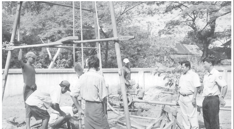
Township DAC sinking a tube well for Taunggyikwe Village in Bago Township.
