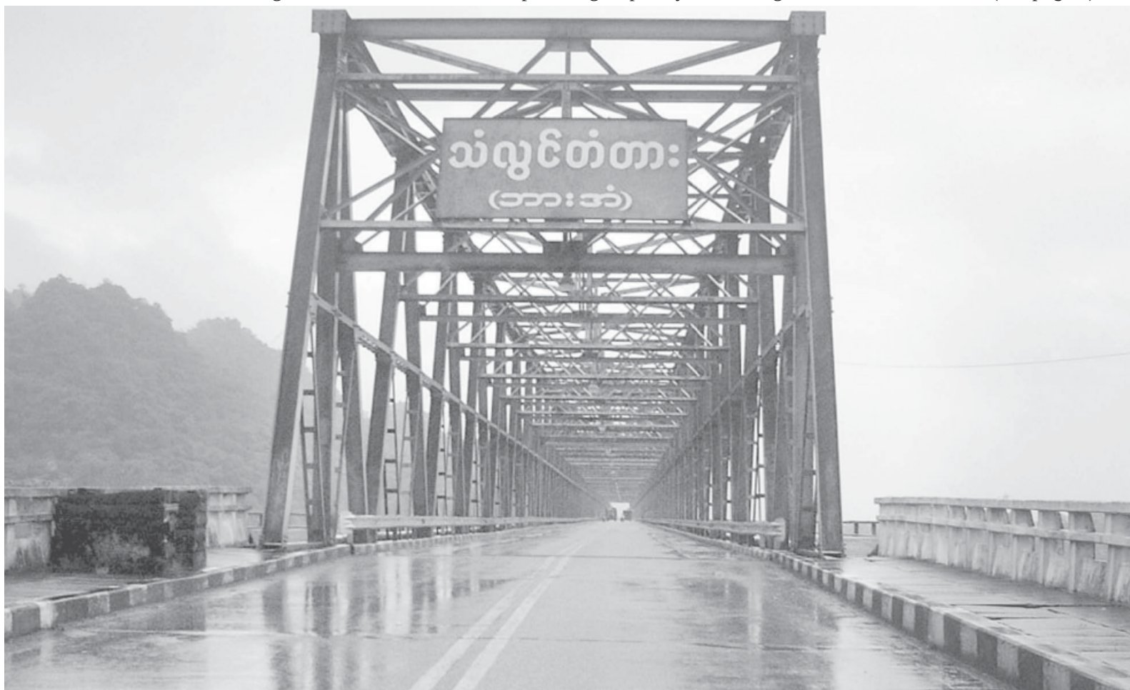
Thanlwin Bridge (Hpa-an) spanning the Thanlwin River.
