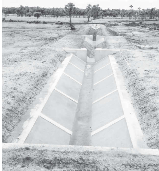
The intake structure of distributary (2) under construction.
