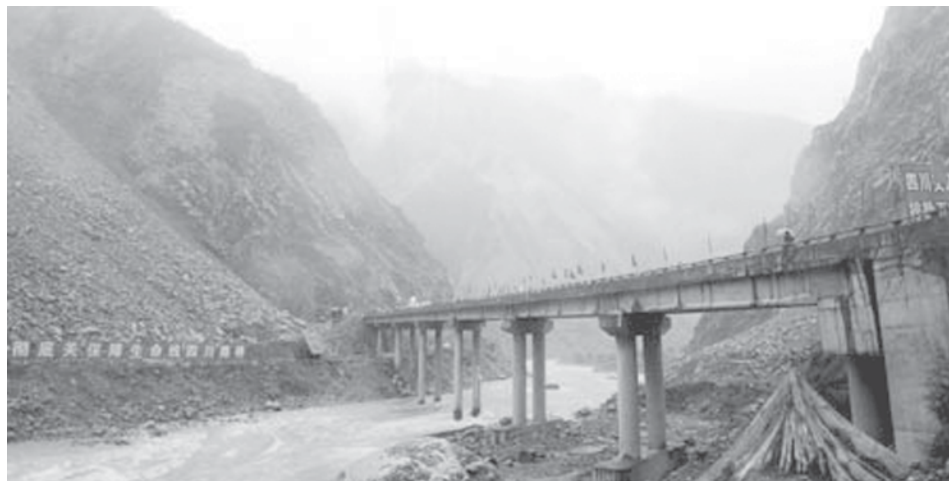
Photo taken on 31 July, 2009 shows the repaired Chediguan Bridge, part of No 213 state highway, in Wenchuan, southwest China's Sichuan Province. The bridge was reopened to traffic on 31 July, seven days after it was damaged by a fallen rock. No 213 state highway is a key traffic line linking Wenchuan County to other areas of Sichuan. —XINHUA
