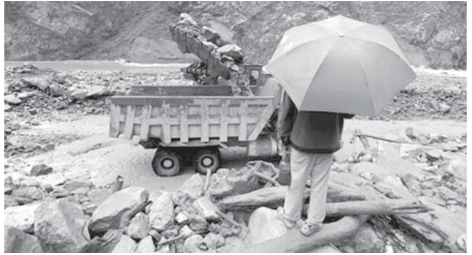
A person watches an excavator working at the site of the landslide in Kangding, southwest China's Sichuan Province, on 26 July, 2009.—INTERNET
