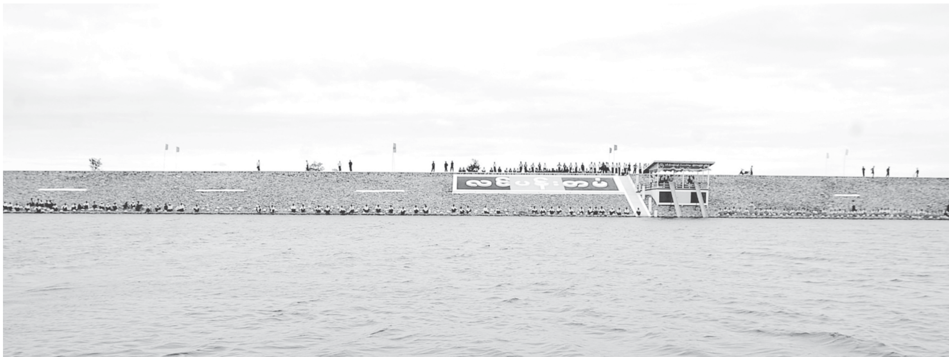
Linpan Dam in Kanbalu Township, Shwebo District, Sagaing Division.—MNA
