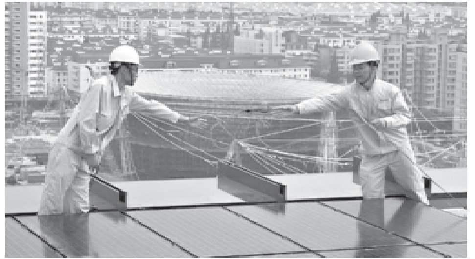
Workers fix solar energy panels on the top floor of the Chinese Pavilion at the Shanghai Expo Site, Shanghai, east China, on 25 July, 2009. 1,264 solar energy panels will be fixed on the top floor of the Chinese Pavilion, which could generate 300 kilowatt-hours of electricity per hour in the sunny days.—XINHUA
