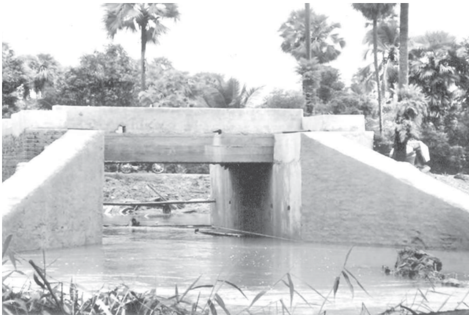
Bridge No (29) in Dawei-Thayetchaung railroad section.
