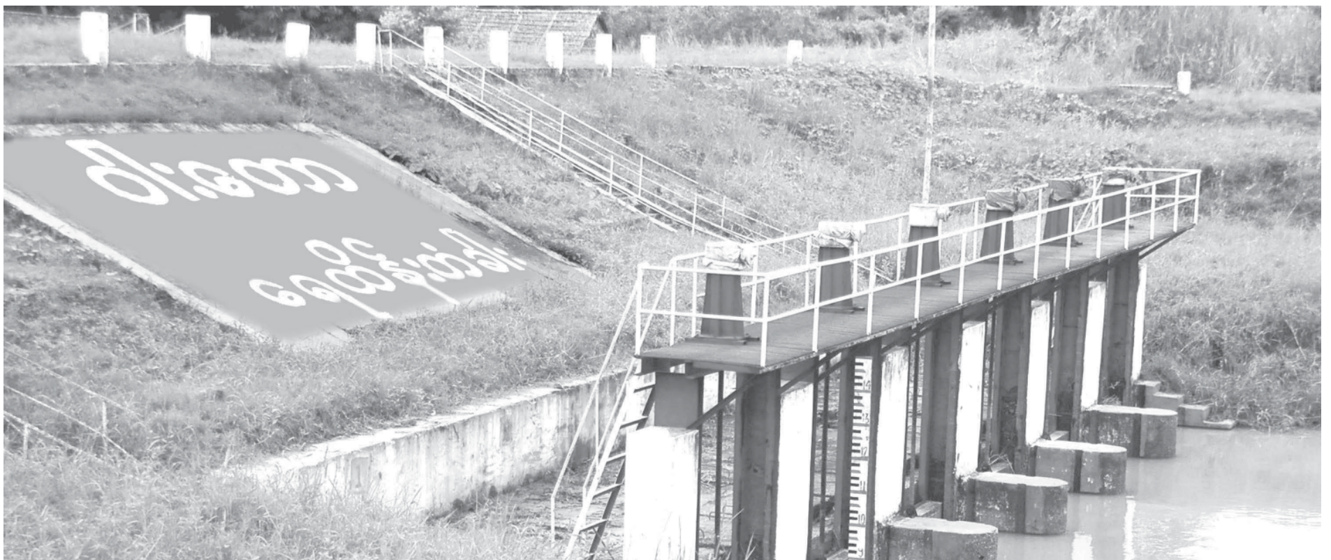
Wadaw Sluice Gate, which benefits more than 10,000 acres of agricultural lands and protects many acres against floods.
