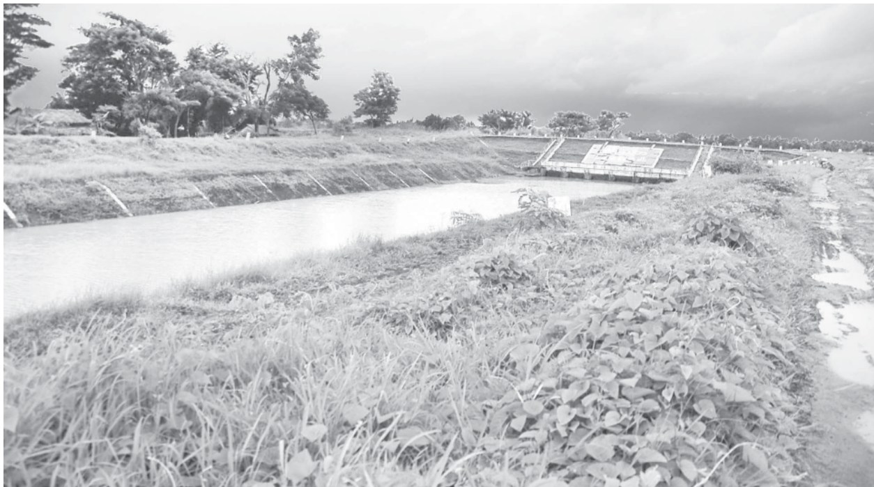
The main canal of Wadaw Sluice Gate in Maubin Township.
