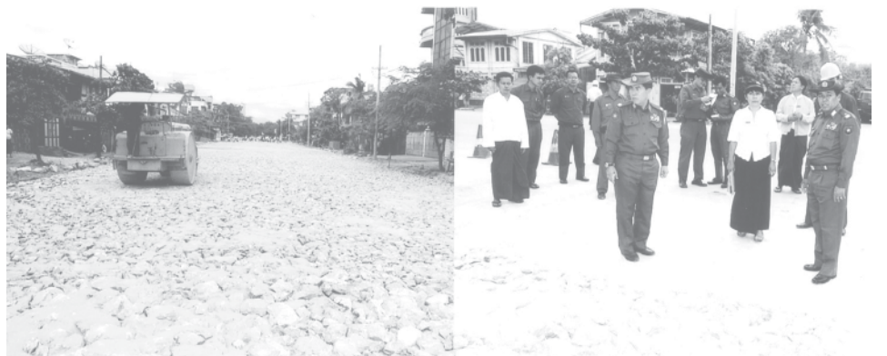
Commander Maj-Gen Tin Ngwe inspects construction of road.—MNA
