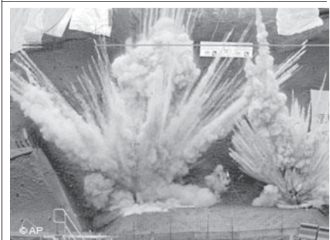
A controlled explosion clears away rock during work on a railway tunnel near the town of Goldisthal in the eastern German state of Thuringia. The tunnel is to be part of a high-speed railway line, currently under construction.
