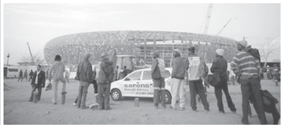
Workers stand outside the under construction Soccer City stadium near Soweto in Johannesburg, June 2009.—INTERNET
