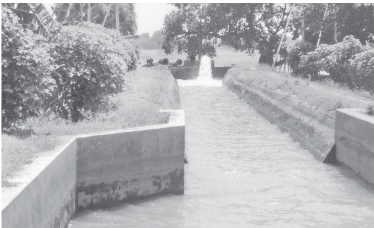
Water is pumped from Chindwin River into the main canal to irrigate farmlands.
