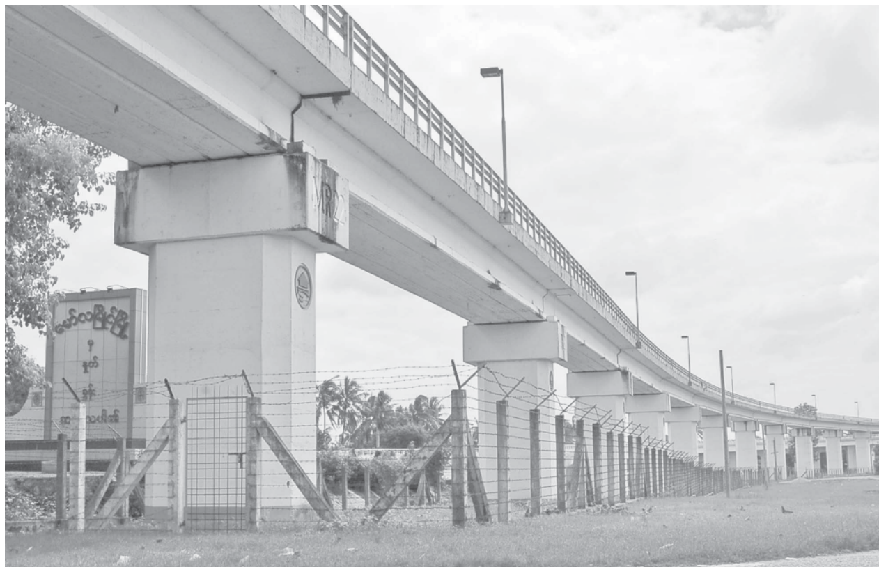
An approach road to Thanlwin Bridge (Mawlamyine).
