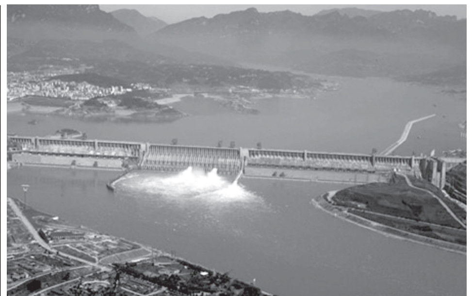
Photo taken on 1 July, 2009 shows the Three Gorges Dam opening two deep-holes and a trash way hole for sluicing the mounting flood water, in Yichang, central China's Hubei Province. The Three Gorges Reservoir has high influx of flooded water along with the arrival of Yangtze River's main flood season with recent days' persistent rainfalls.—INTERNET
