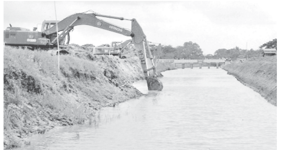
An excavator at work at Thakala-Kayan section.
