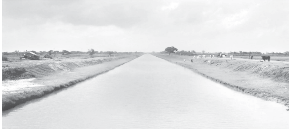
The canal is now filled with rainwater.
