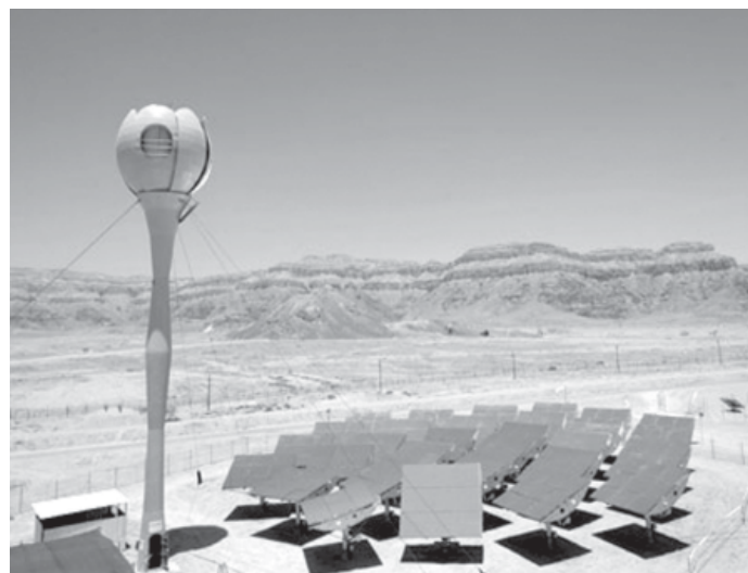
Photo taken on 24 June, 2009 shows the solar receiver of the world's first hybrid solar thermal gas turbine power station at Kibbutz Samar in southern Israel. XINHUA
