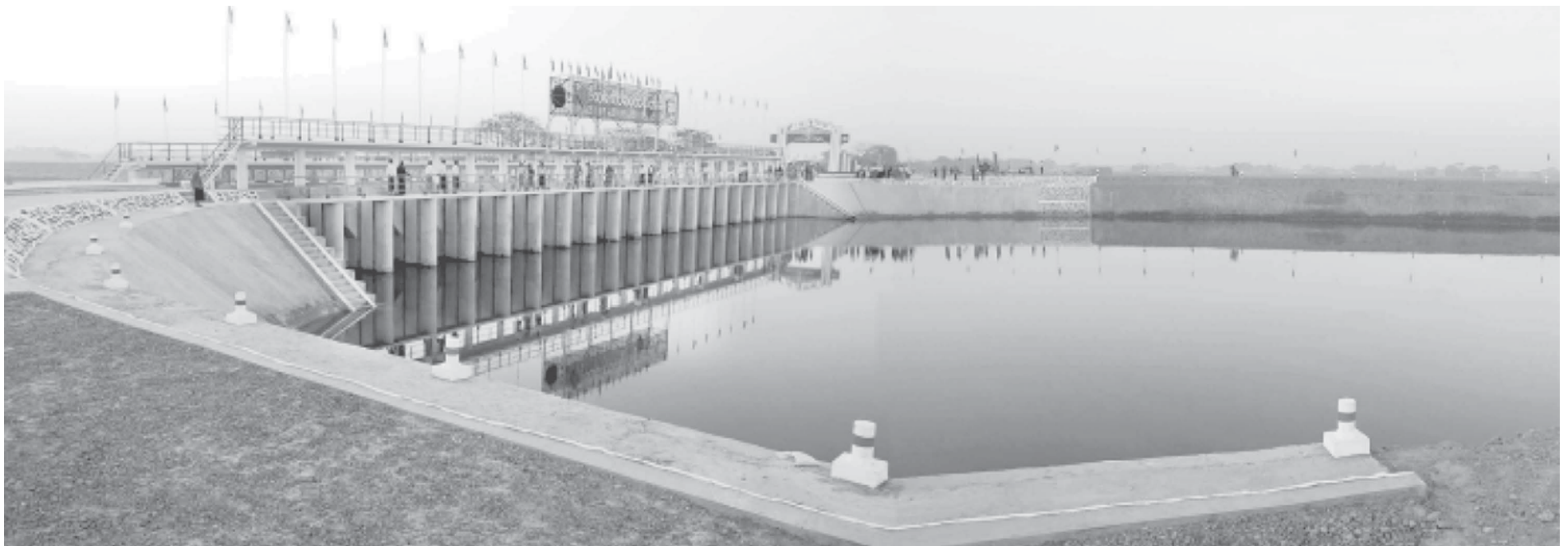
Takaw Sluice Gate stores water from Takaw Creek in Thongwa Township.
