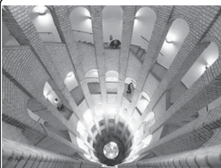
After three years of renovation, the French Cathedral at the Gendarmenmarkt in Berlin reopened. It now has a viewing platform - at the top of this staircase - which is opened to the public.
