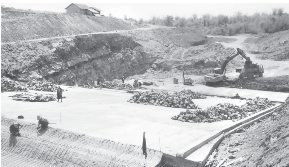
The 220 feet long and 100 feet wide spillway is under construction.
