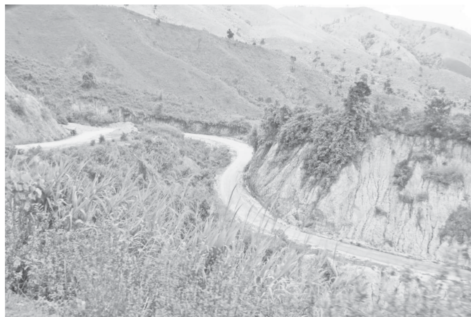
Kengtung-Taunggyi Road seen on hilly area.
