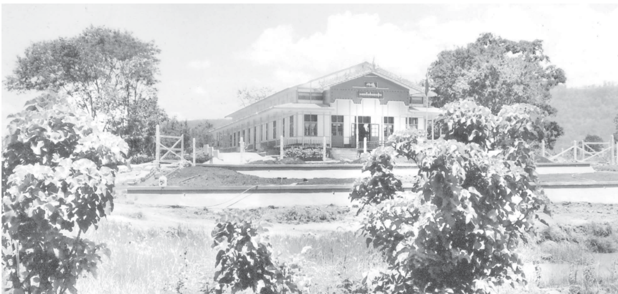
Hsenwi Town Hall is under construction.
