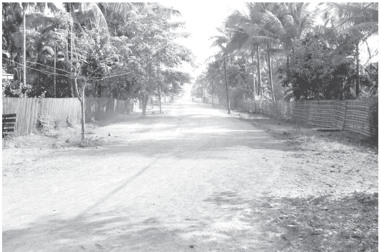
U Uttama Road seen after being renovated.
