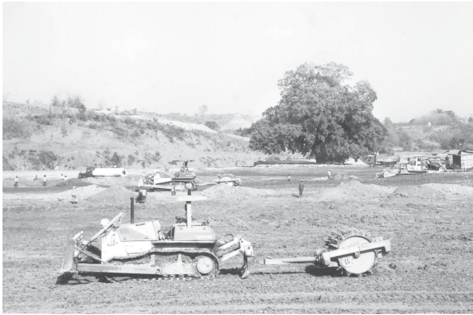
Groundwork is done with heavy machinery.
