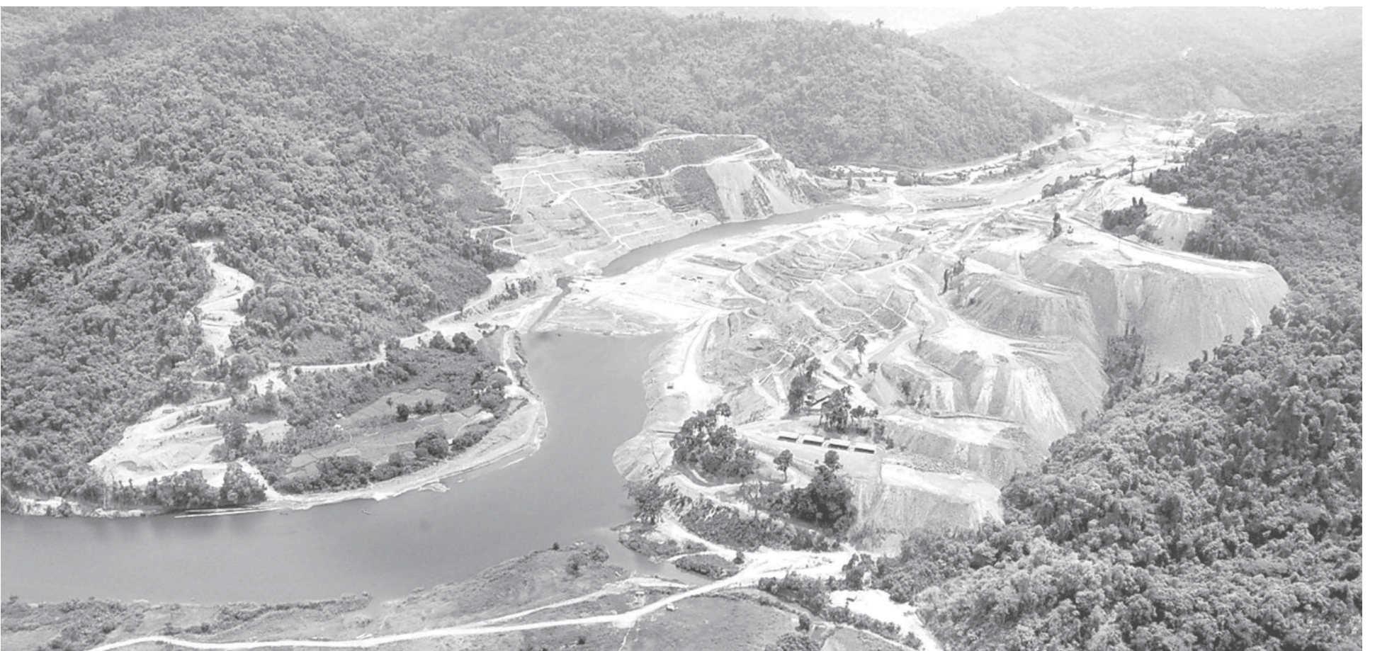
Thahtay Hydro Power Project Site.—MNA
