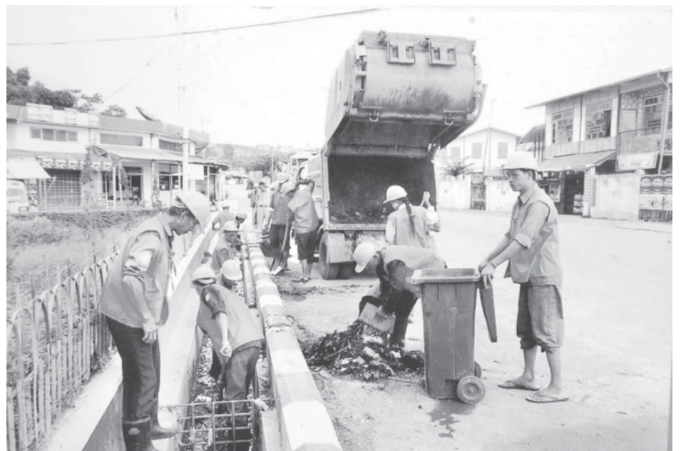
Workers dredging a drain in downtown Taunggyi.
