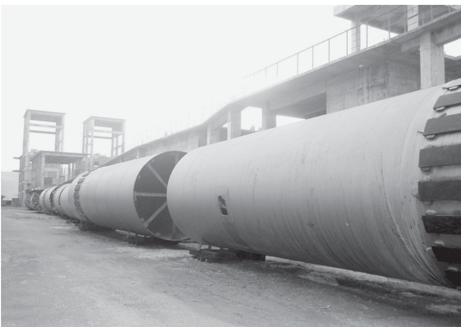
Naga cement plant (Tikyit) project is under inspection.—MNA
