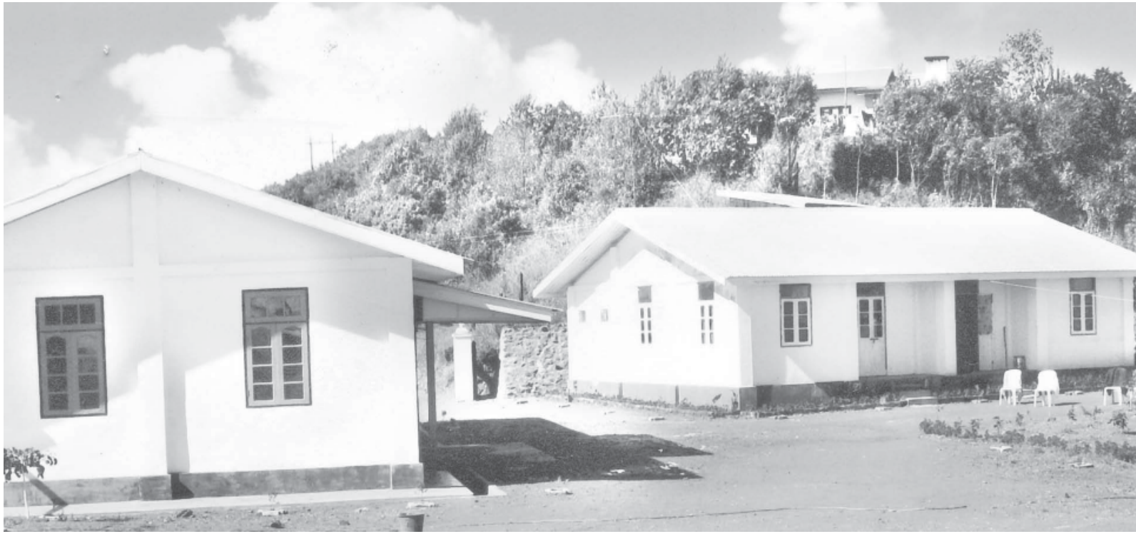
One storey hostel for trainees.
